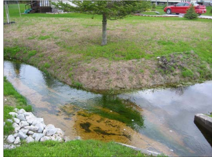
Unstable streambank on north side of M-134
